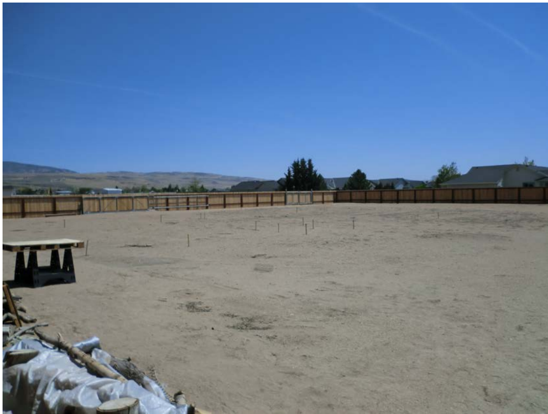
The rear yard where the accessory structure will be built. The footprint of the structure is staked out in the yard.
